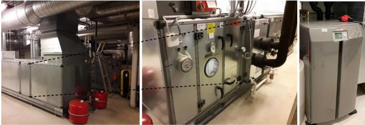
**Figure 5: Exhaust air unit of washrooms and dressing rooms from different sides, additional heat exchanger installed (dashed lines indicate location); heat pump Gebwell T2 (right)**
